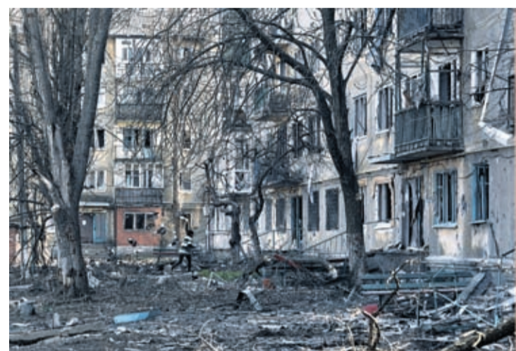
A local resident runs past the damaged houses in Bakhmut, the site of heavy battles with Russian troops in the Donetsk region, Ukraine, Sunday, Apr. 9, 2023.
